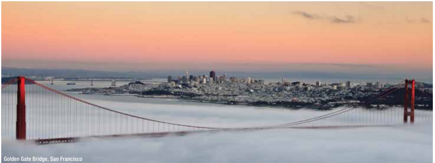
Golden Gate Bridge, San Francisco
